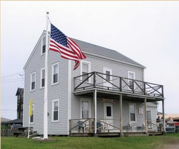
Current NSWFC Clubhouse after repairs & renovations
